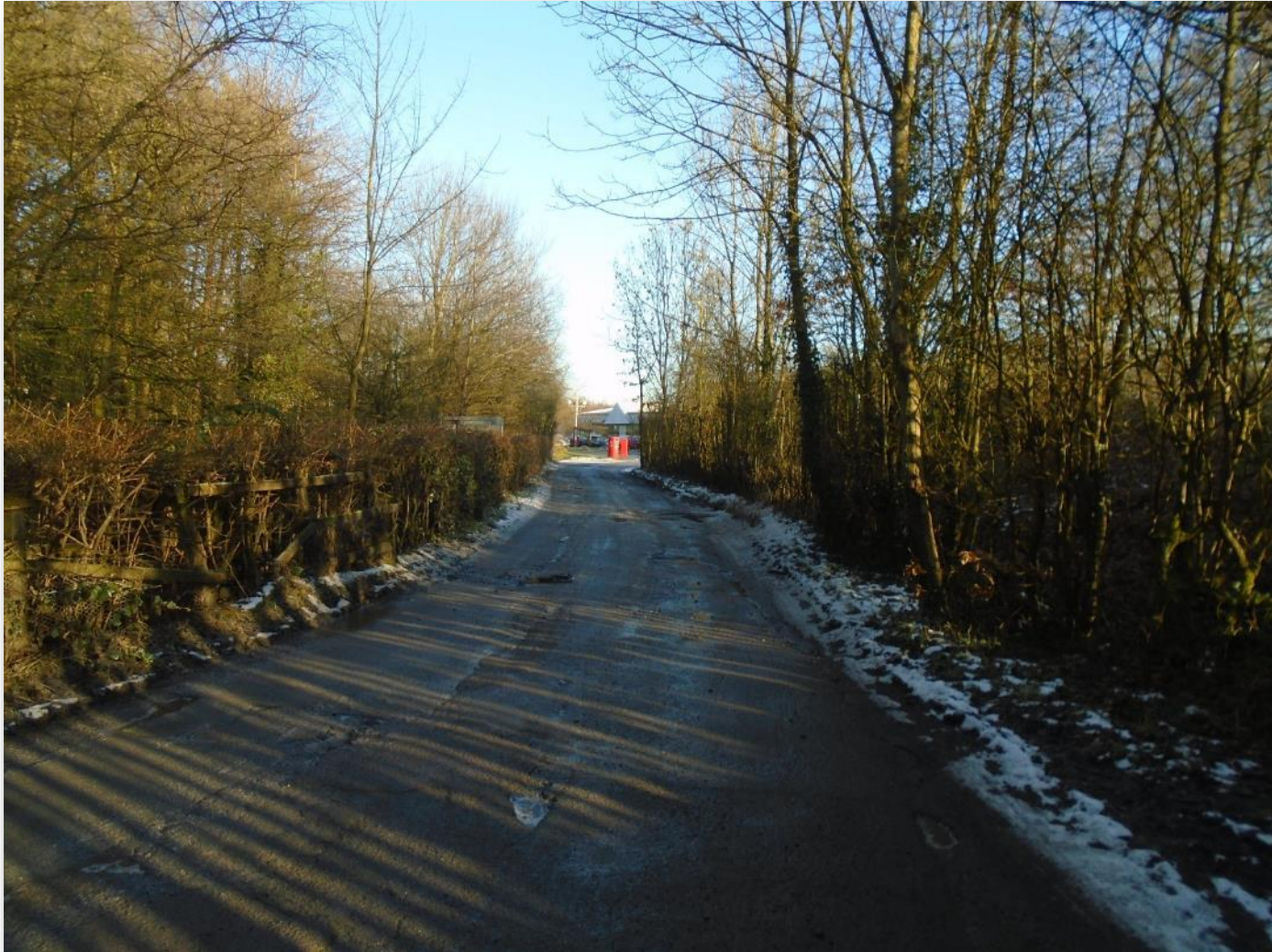
Common Bank Lane towards the junction with Ackhurst Road
