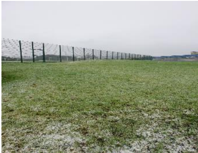
Existing MUGA Fencing
